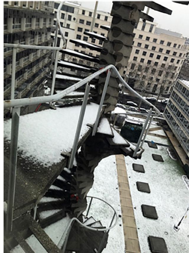
A precarious-looking exit stair (no longer the primary means of emergency egress) at Breuer, Nervi, and Zehruss' UNESCO Headquarters Paris, 1958; photograph by the author, January 2019.
